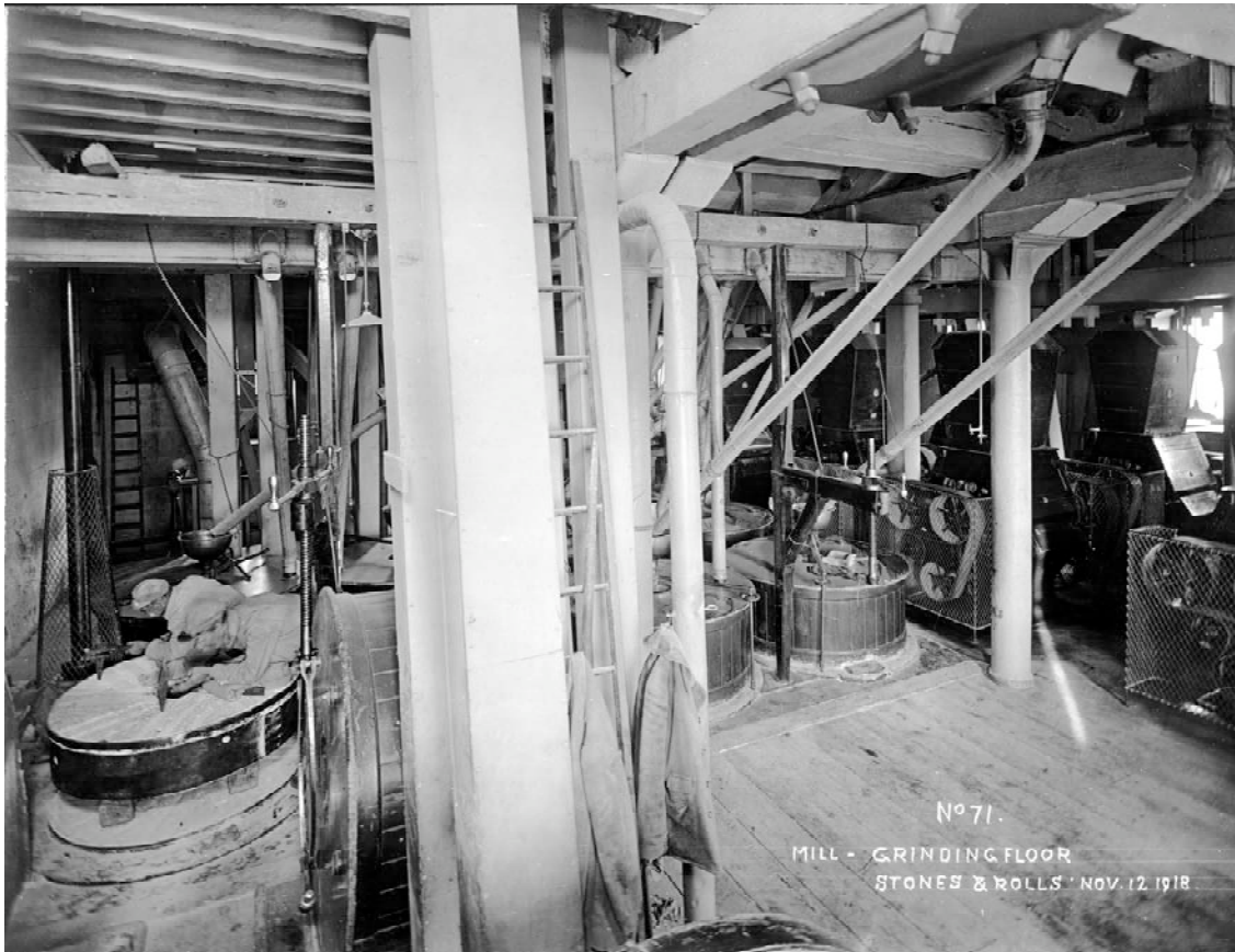
1918 Mill floor with millstones & high rollers
