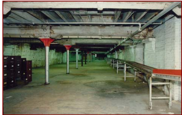
Building 58 2 nd floor storage & old conveyor
