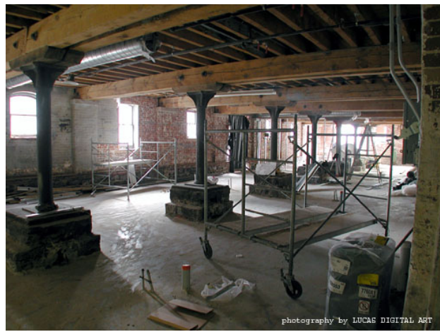
New floor & sand-blasted walls Thane Lucas
