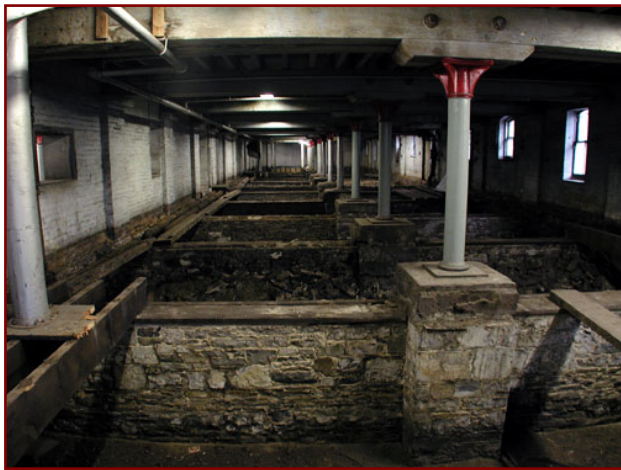
Cannery wood floor removed Thane Lucas
