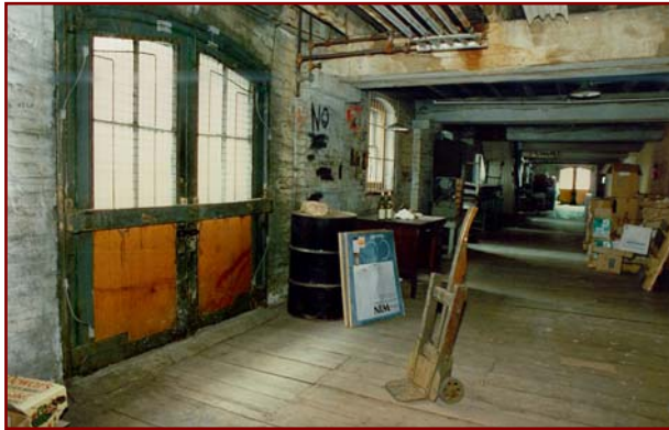
Building 59 1 st floor looking toward Trinity St.
