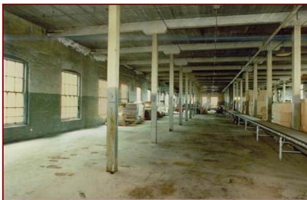
Building 58 & 59 3 rd canning floor
