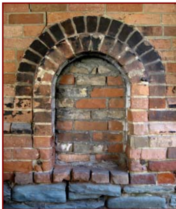
Exterior stoking hole
