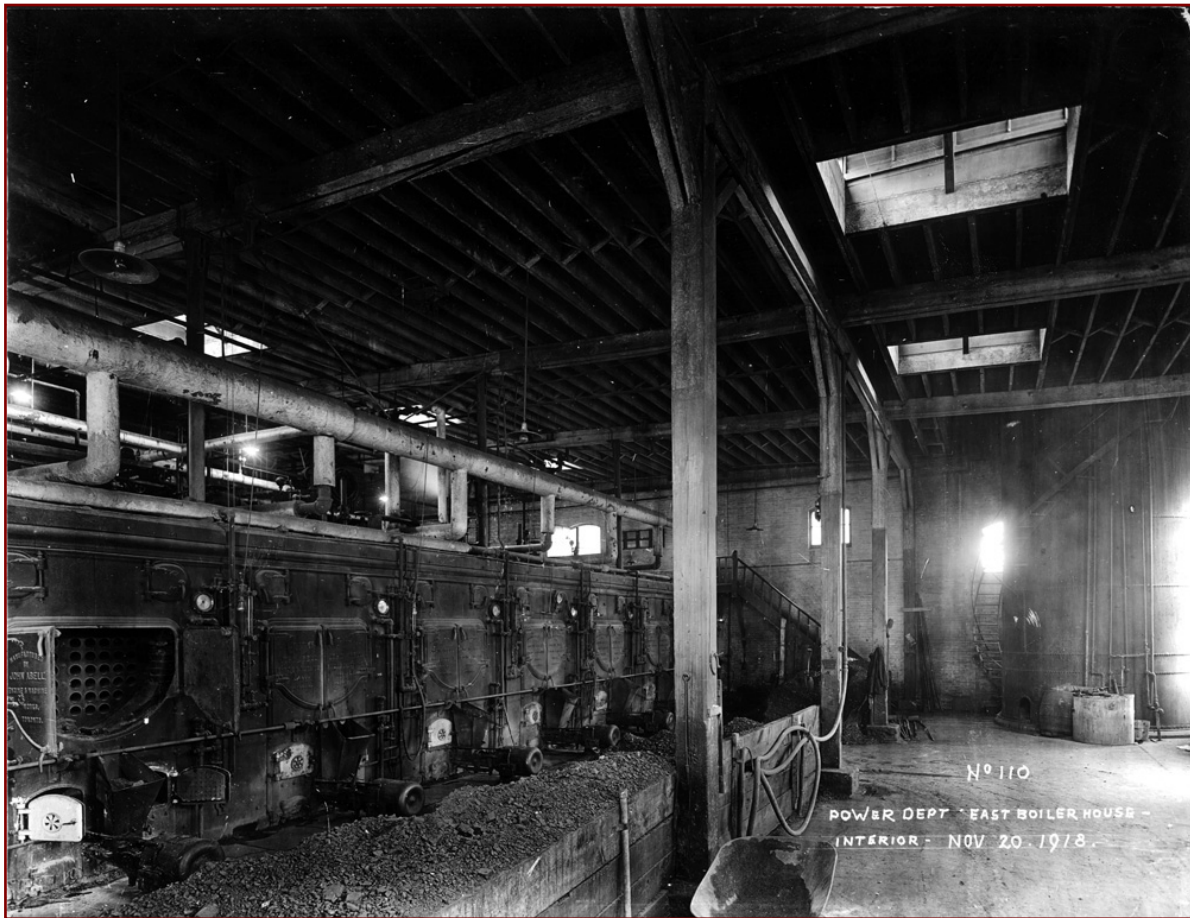
Building 46, looking north along battery of eight Abell boilers, 1918 CTA 1583-110
