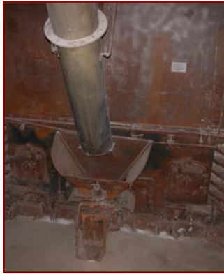
Automatic coal-stoker at base of boiler
