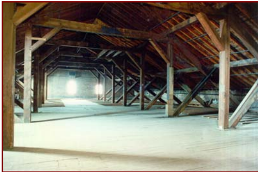
Building 35, empty attic
