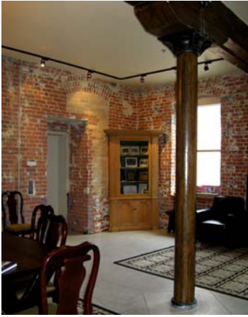
Building 32: school library cabinet, column & double timber beams
