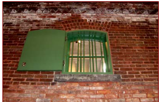
Window in west wall of Building 50
