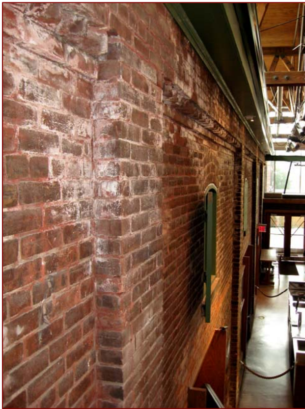
Looking south along east wall of atrium
