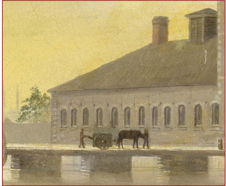
South side of reconstructed Fermenting Cellar, 1870 DHD
