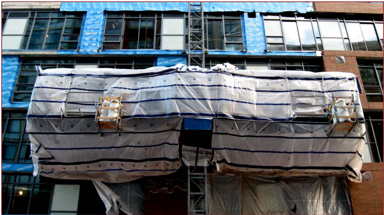
Bricklaying at about 20-below
