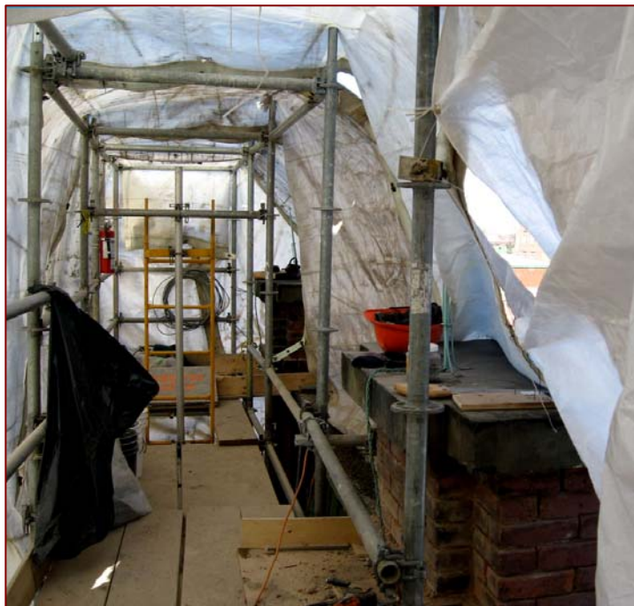
Undercover operations atop Buildings 53-57
