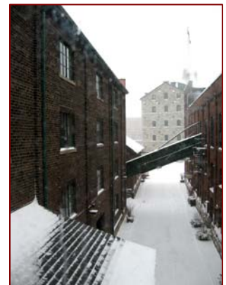
From 3 rd floor bridge
