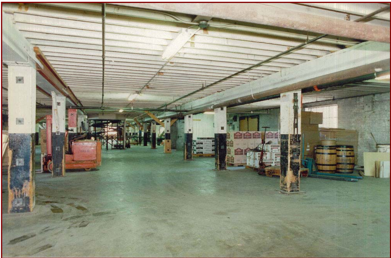
Case Goods Warehouse, 1 st floor looking west toward spiral slide in the distance Larry Turner
