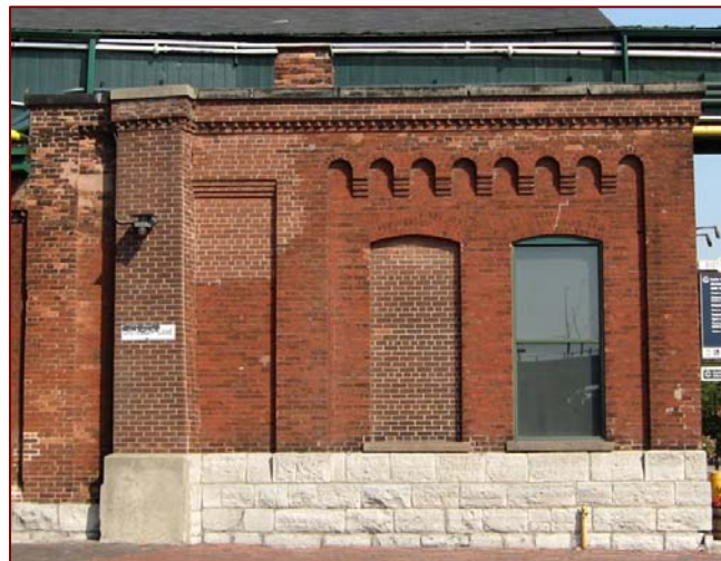
South façade of Building 31 today
