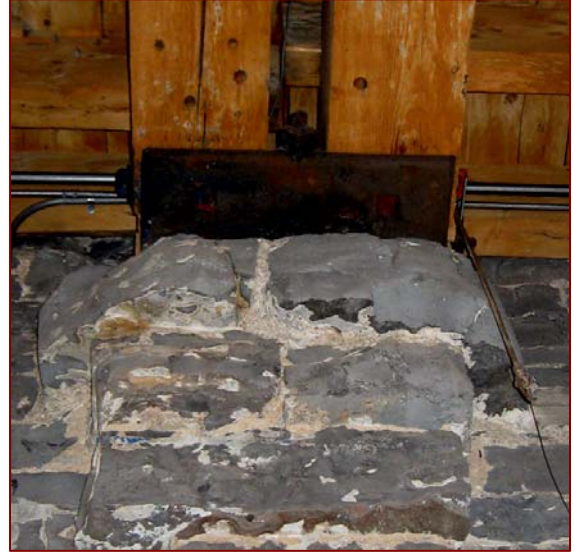
Stone Distillery double beams on limestone corbel
