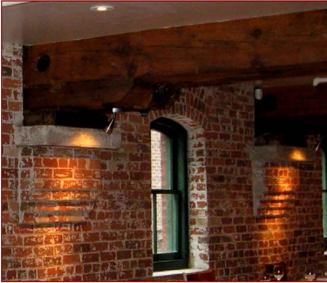
Cannery double beams on stone & brick corbels
