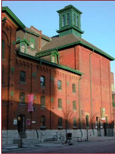
No tie plates on Kiln Building
