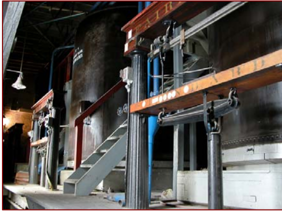
Scale tanks with capacity of 25, 210 litres
