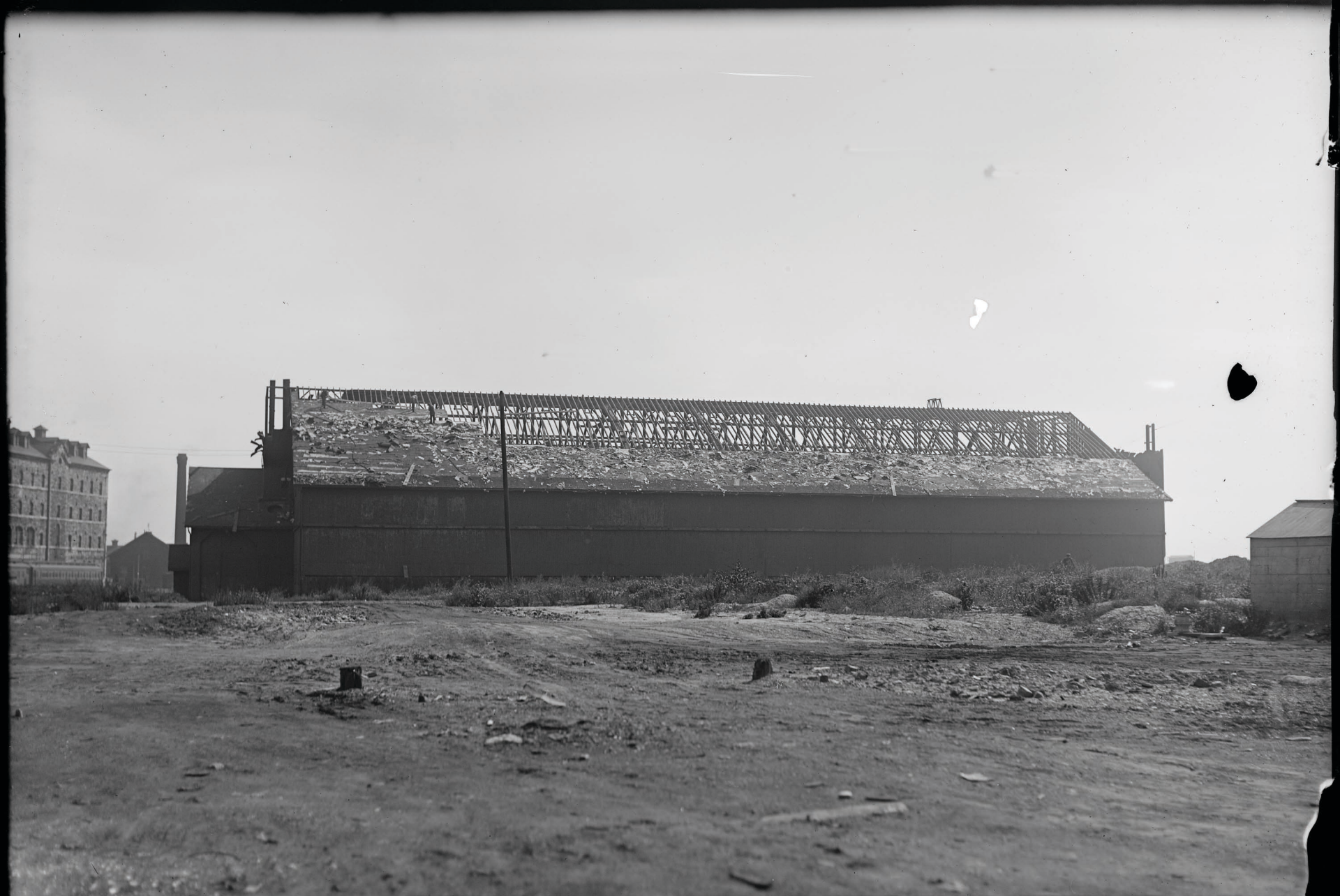
VIA 85. SEPT 2-1926. GOODERHAM AND WORTS ELEVATOR.
