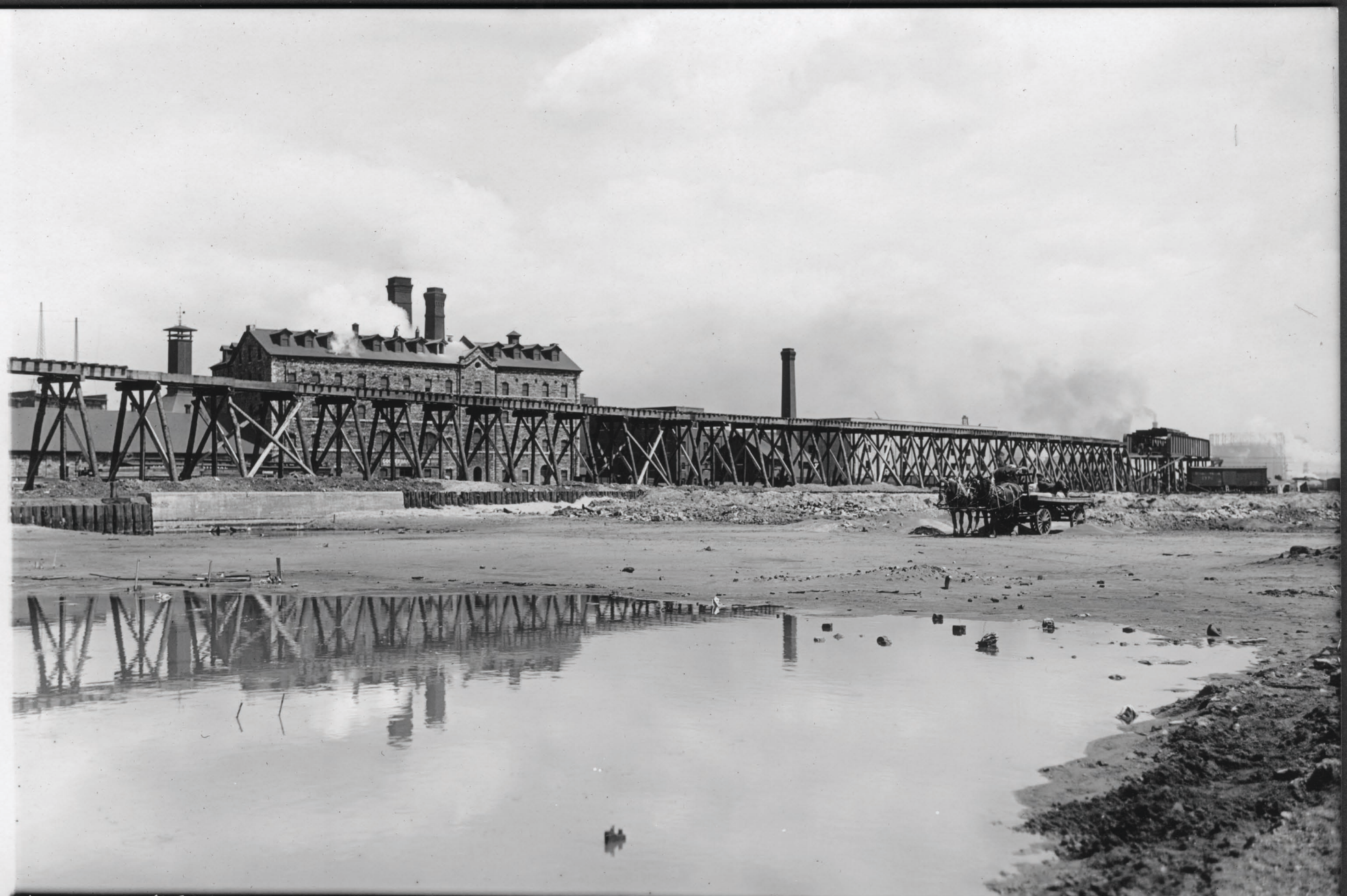
VIA 209. APR 28-1927. TRESTLE EAST OF PARLIAMENT. ST.
