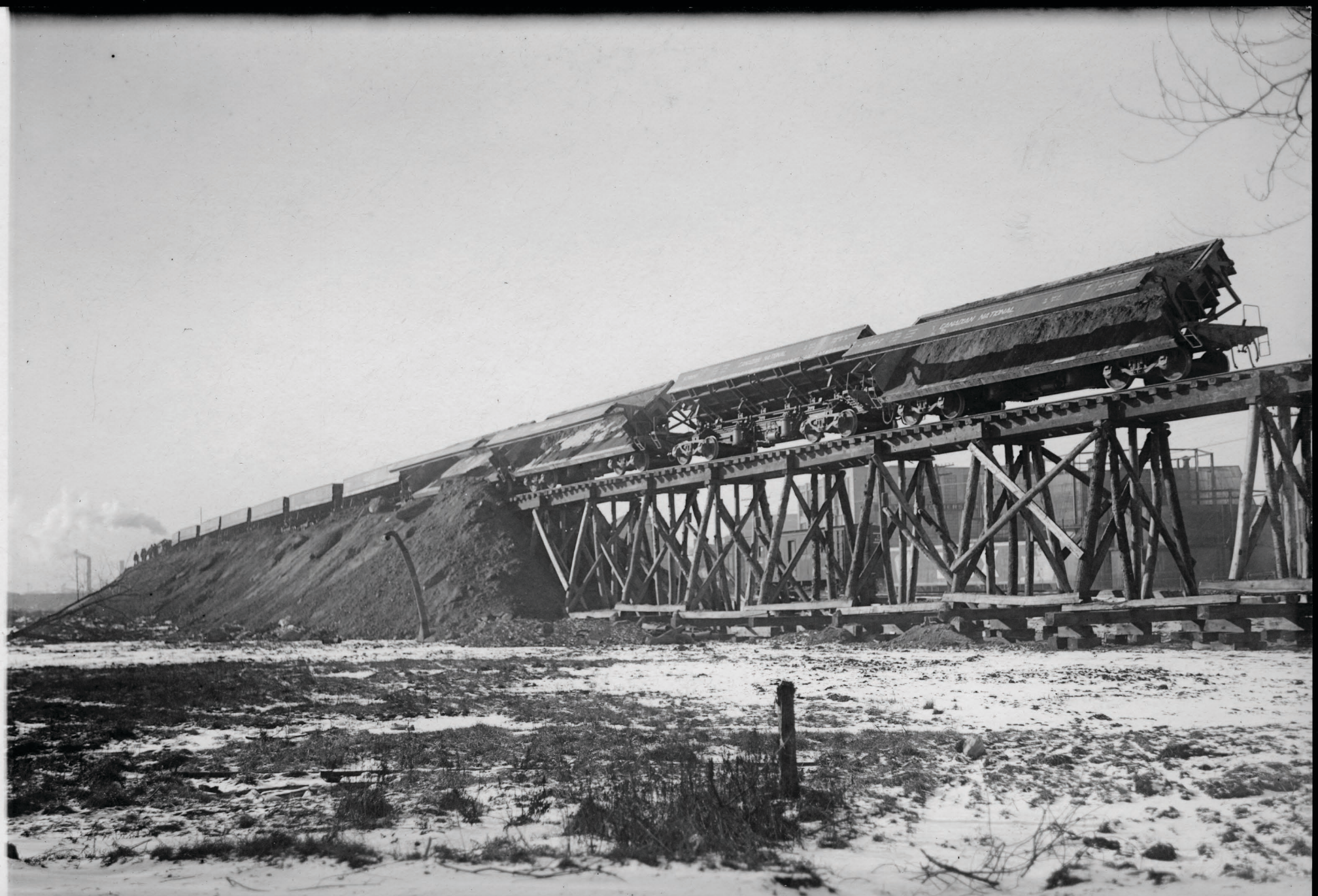
VIA 179, JAN 5-1927, WEST OF EASTERN, FILLING TRESTLE.
