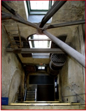
Looking down 3 storeys
